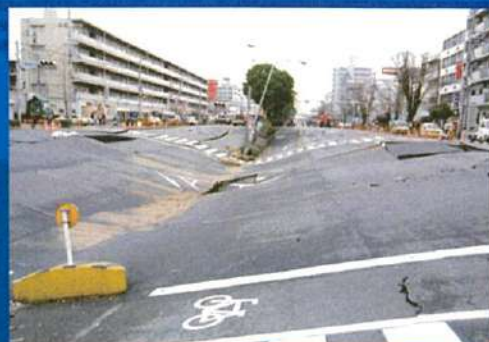
道路の陥没、国道28号線、地下に神戸高速鉄道 大開駅がある付近 神戸市長瀬区 1995.1.23 Caved in road, National Highway Route No. 28, near Daikai Station on the underground Kobe Rapid Transit Railway, Higashi Ward, Kobe City. 23 January 1995.
