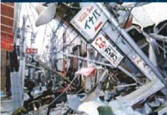
三宮の電柱。電柱が倒れ店のインテリアが道路に散乱 神戸市中央区 1995.1.23 Damage to Chiba Towers in Sannomiya. Electricity poles have fallen and the shop interiors are spilling onto the street. Chuo Ward, Kobe City. 23 January 1995.
