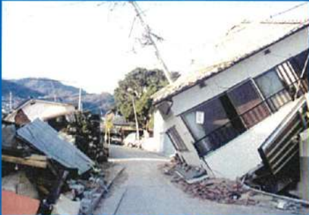
2階部分の一边が地上に落ちるほど傾いた住宅。背景には、同じ方向に傾いた電柱と別の住宅が見える。地震動の力のかかった方向がうかがえる 丹波市 1995.2.21 Part of the second floor of this house is touching the ground. An electricity pole and another house, also tilting in the same direction, can also be seen, showing the strength of the earthquake and the direction of its force. Aishiya City. 21 February 1995.
