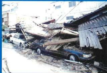
木造家屋が全壊し、車の上のしかかっている 丹波市 1995.2.21 Wooden house is totally destroyed and has fallen on top of parked cars. Aishiya City. 21 February 1995.
