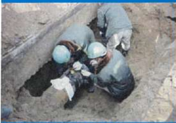
ガスの復旧作業に全国の一般ガス事業者の応援隊が駆けつけた Supporters from general gas companies around the country came to restore gas infrastructure.
