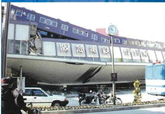
駅舎の1階エントランス部分がつぶれた阪急伊丹駅 伊丹市 1995.1.17 Izumi Station on the Hankyu Line. The ground floor entrance has collapsed. Izumi City. 17 January 1995.
