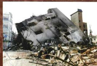
地震で倒壊し、その後の火災で燃えたビル 神戸市長田区 1995.1.28 Building that collapsed in the earthquake and was burnt in the resulting fires. Nagata Ward, Kobe City. 28 January 1995.
